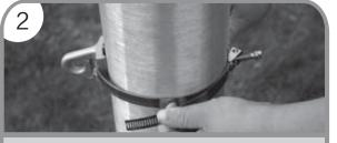
2. Determine the location of the bottom of the banner. Wrap the Steel band (G) through the Eyelet bracket (H) and adjust around the pole. Pull the Steel band (G) tight and secure the screw locking-mechanism by pushing down.
