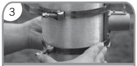
3. Place the Mounting bracket (C) between the Steel band (G) and the pole. Pull the Steel band (G) tight and secure the screw locking-mechanism by pushing down. Repeat Steps 2 and 3 for the second Steel band (G) on the top Mounting Bracket (C).
